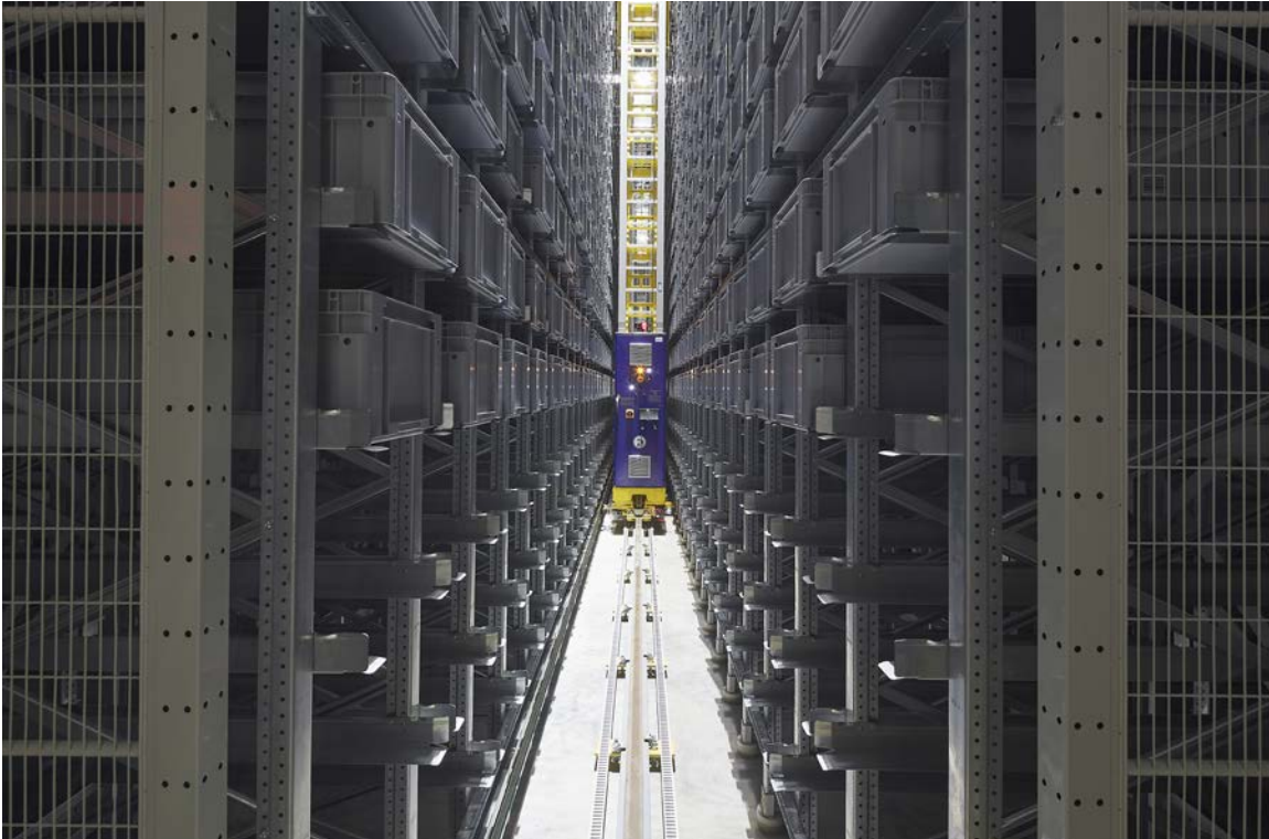
Figure 4 The ASRS warehouse of the Kooperative Speicherbibliothek Schweiz. Photo: Ulrich Niederer
