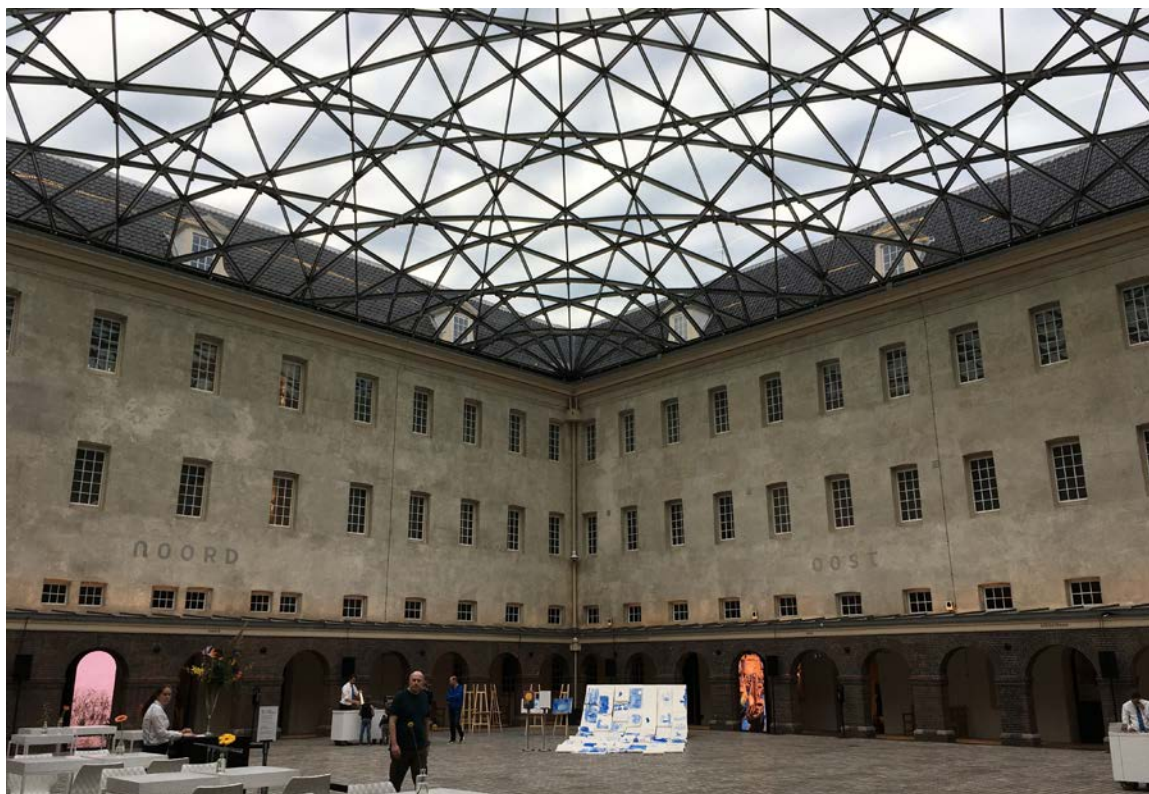
Figure 8 Roof canopy over the National Maritime Museum inner courtyard. Photo: Agnes Brokerhof
